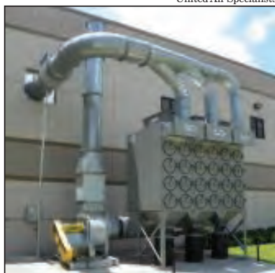
FIGURE 1. Reputable air-pollution-control experts can recommend appropriate systems like United Air Specialists' SFC cartridge dust collector, which can be equipped and installed to safely handle hazardous dusts
